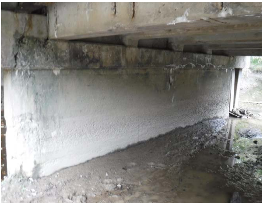
FRONT OF PIER
