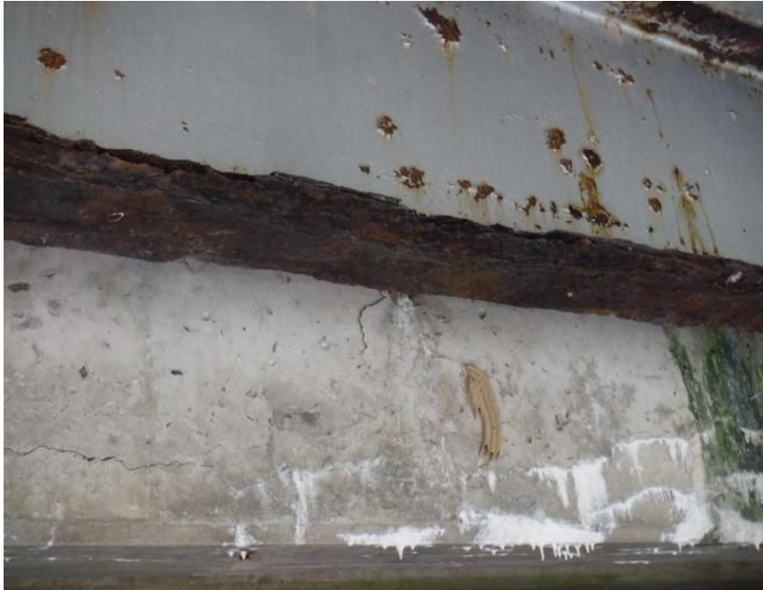
SPAN 1 BEAM "B"
