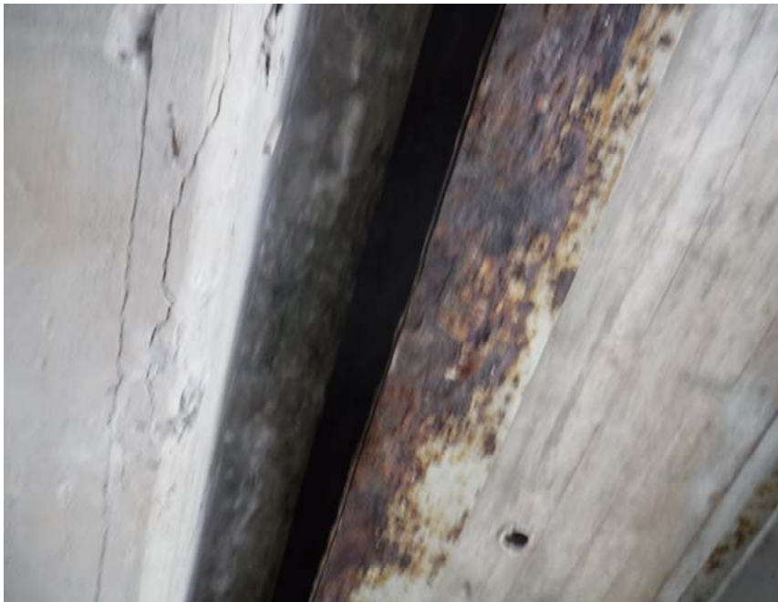
SPAN 2 BEAM "H"
