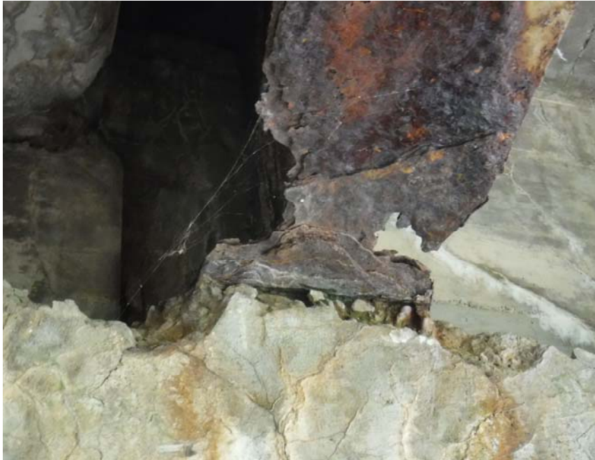
SPAN 2 BEAM "H"
