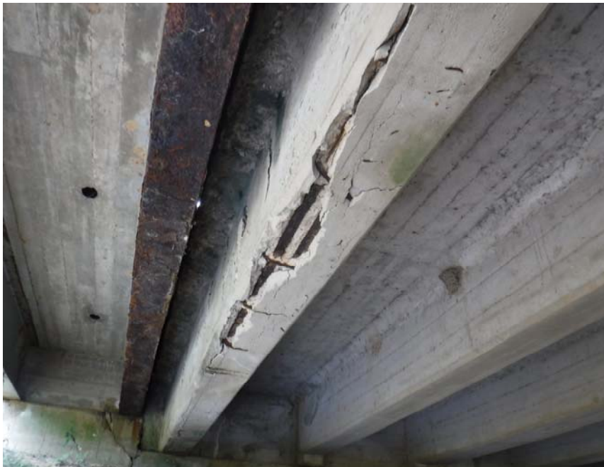
SPAN 2 BEAM "B"
