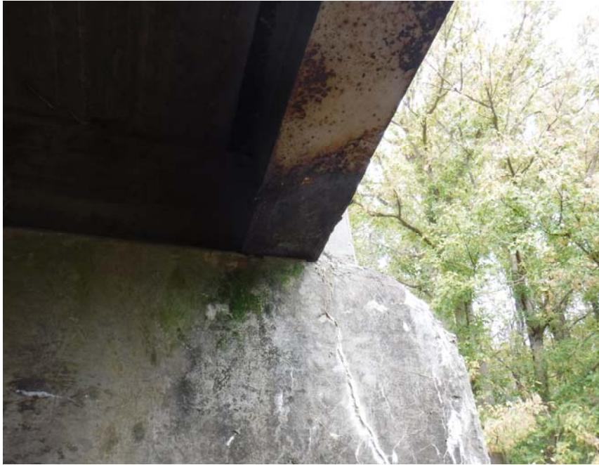
SPAN 1 BEAM "I"
