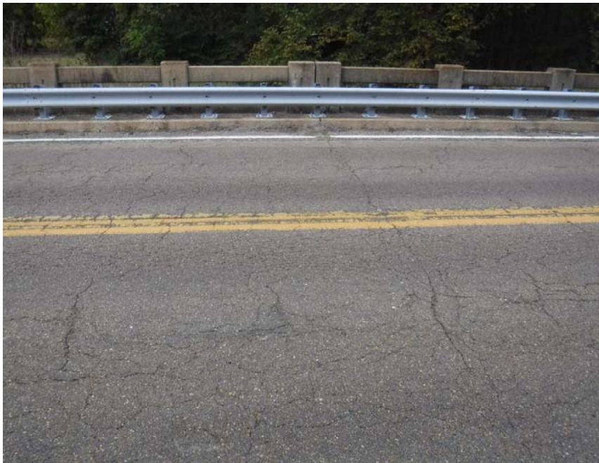
VIEW ACROSS TOP OF DECK
