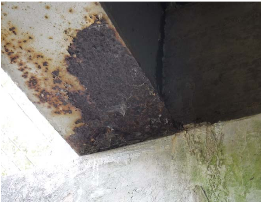
SPAN 1 BEAM "A"
